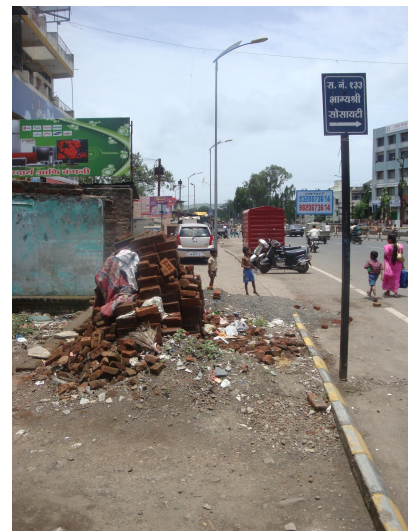
Picture 3.5.3: Construction material on Cycle Track
