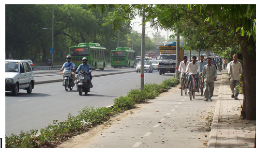
Illustration 4: Well designed cycle tracks along the Delhi BRT corridor are free from obstructions and have a smooth riding surface.
