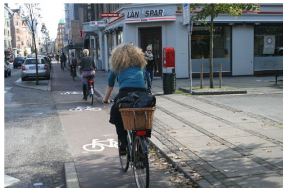
Illustration 3: Where cycle tracks are not segregated they can still be well marked so as to maintain visual continuity for cyclists.
