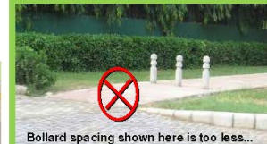
Bollard spacing shown here is too less...
