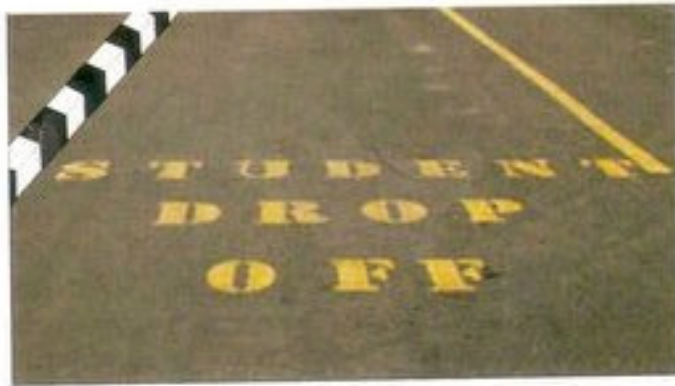
Photo 15 Marking of Student Drop off Area
