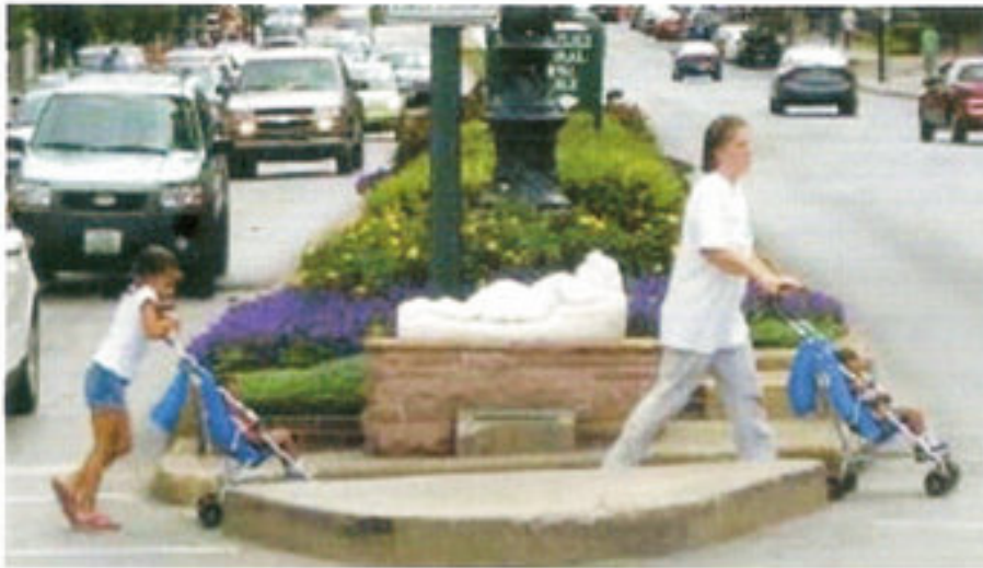
Photo 8 Median Pedestrian Refuge on Two-Way Road
