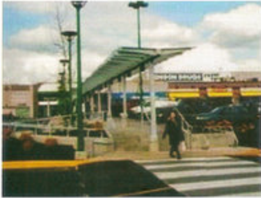
Photo 18 Pedestrian Facilities at Transit Area
