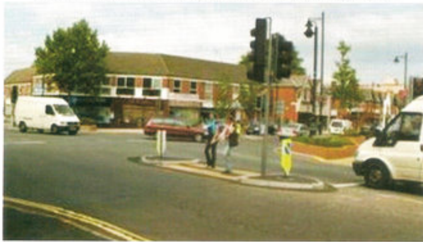
Photo 9 Median Pedestrian Refuge at Signal-Controlled Junction
