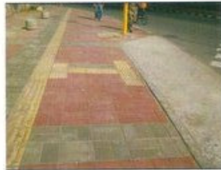
Photo 5 Tactile Paving on Footpath Leading to Ramp and Crossing
